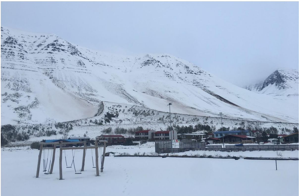
Figure 2.4: Photograph of the avalanche barrier in Flateyri. The barrier protects the residential area that was hit in 1995 causing 20 deaths (photograph by author)
