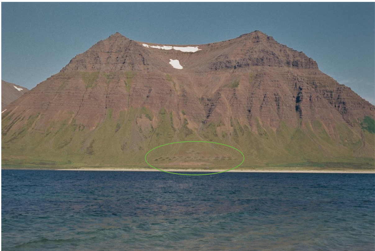
Figure 2.3: Photograph of avalanche barriers protecting infrastructure. In the centre of the image (below the large bowl-shaped depression and main gully) are two rows of vegetation-covered mounds designed to break up the avalanche flow. They are built to protect the road to Flateyri below. Avalanche and debris run-off mounds can be discerned below almost all of the smaller gullies (photograph by author).
